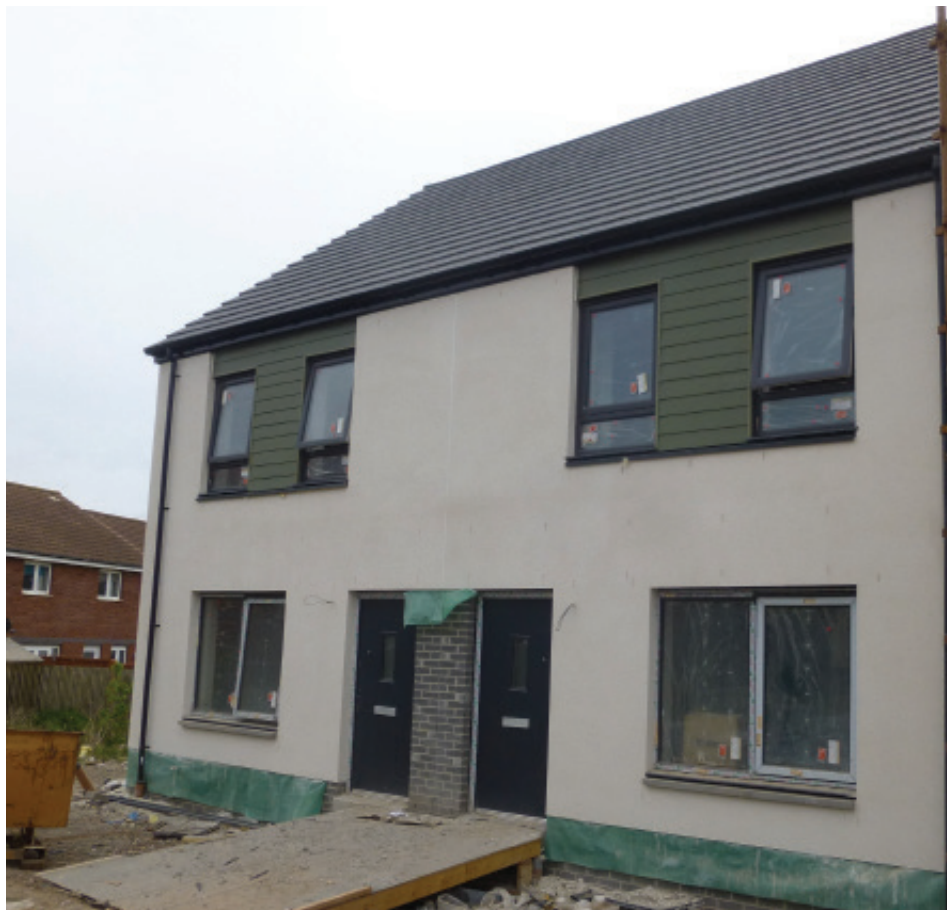
Work is progressing well at Acredale, Eyemouth
